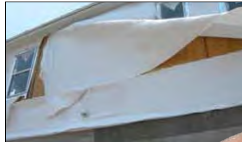
Traditional mechanically fastened wraps may shed water, but fully bonded BlueskinVP provides impenetrable protection against air and water.
