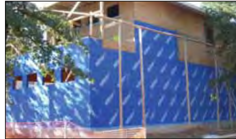
BlueskinVP provides a continuous plane of air-tightness to block the movement of air and moisture.
